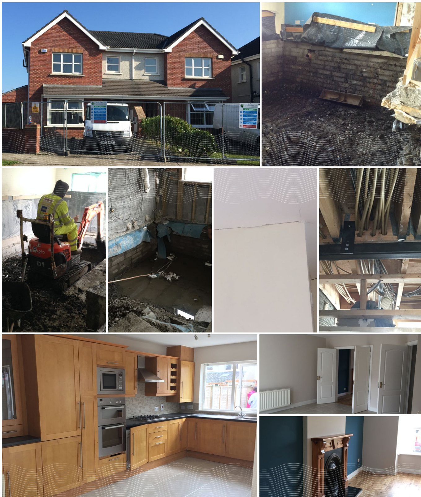
Pyrite remediation work in 2015
